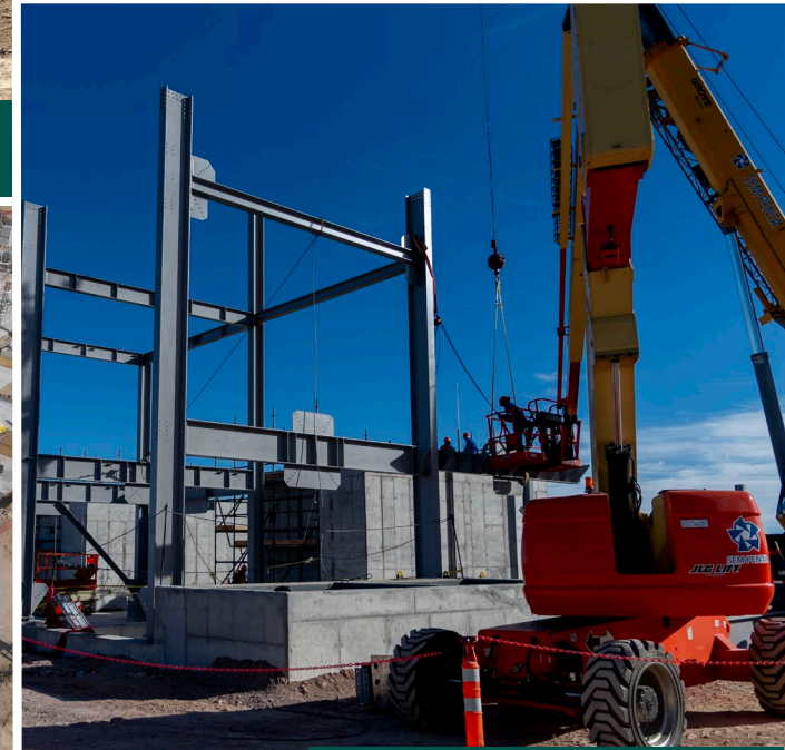
Mill platform structural steel
