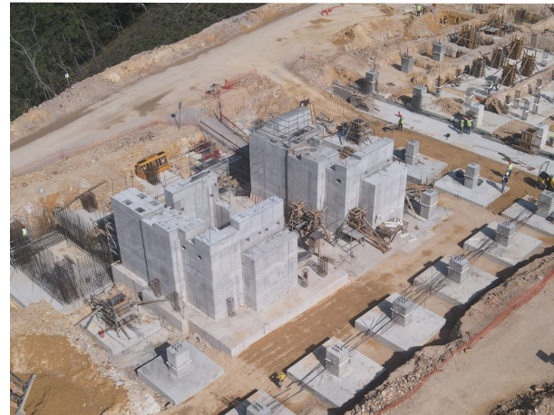
Grinding area ready for mechanical installation
