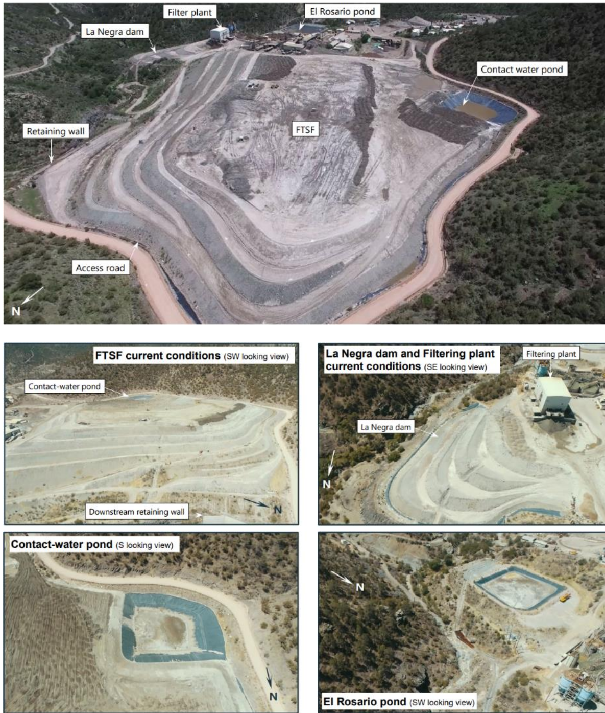
Figure 18-5: Aerial Views of the Plant and Tailings Facilities showing all main features including Contact Water storage
